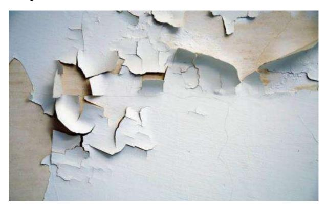
Water beads on the walls or any surface for prolonged periods can cause paint to start peeling.
