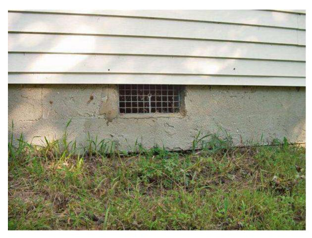
If not adequately ventilated, a crawlspace can quickly accumulate moisture. Depending on the home, a crawlspace may be completely enclosed, sealing any humidity. Installing a wall vent can help improve airflow through the area, preventing moisture from getting trapped. Homeowners can also install an exhaust fan to help remove high humidity during the warmer months.
